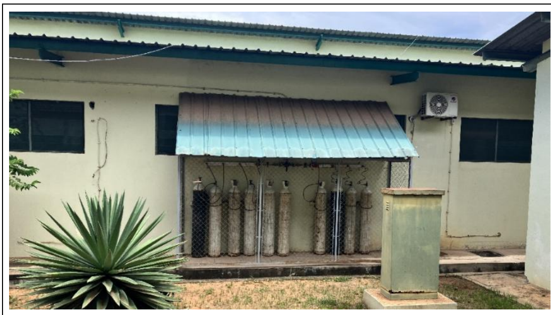
Figure 2: Current Oxygen Manifold for ICU.
